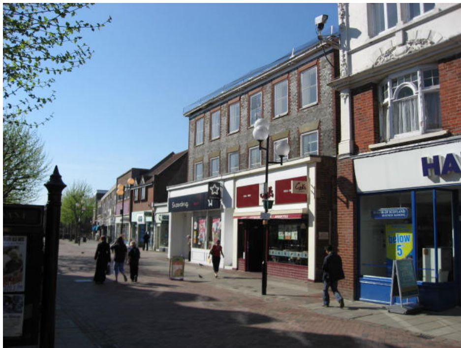
Figure 68: Shopfront does not respect the architectural integrity of the host building (Nos. 28-30 West Street)
