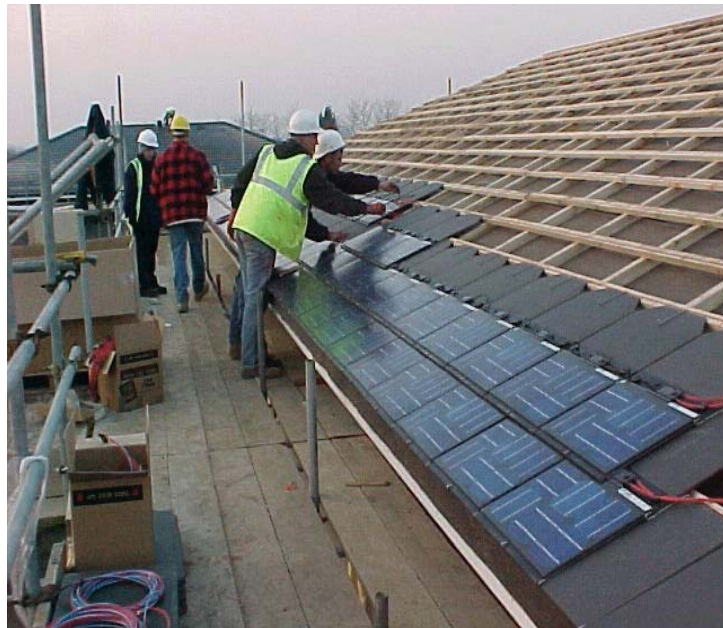
Installation of solar photovoltaic sunslates
