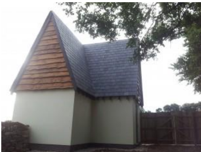
Photo 1: Purpose built bat house designed by EAD Ecology for Cavanna Homes development at Torbay includes features suitable for rare horseshoe bats and was completed in spring 2013
