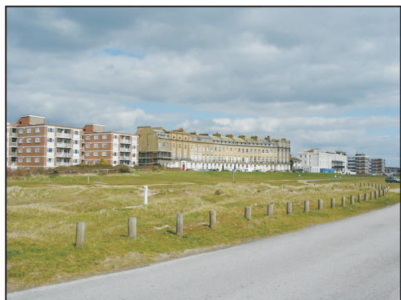
Norfolk Crescent from the south-west
